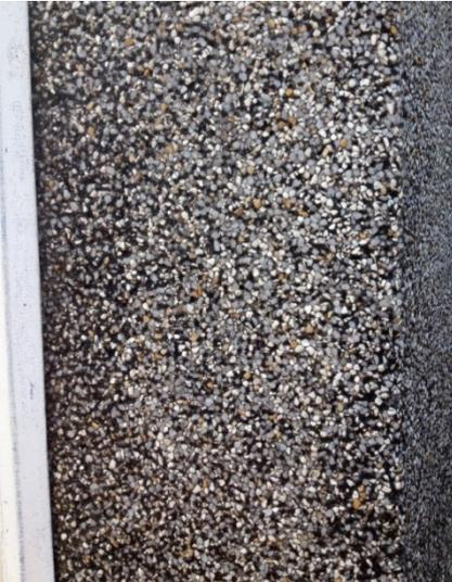
Figure 1: Close up of trowelled surface finish
