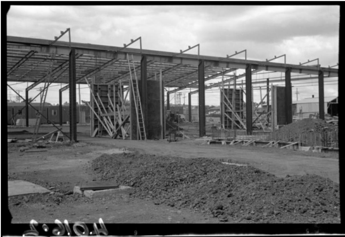
A new building under construction for New Lynn's shopping mall showing the girder framework structure, November 1969. Image: J. T. Diamond Collection JTD-11A-04016-2
