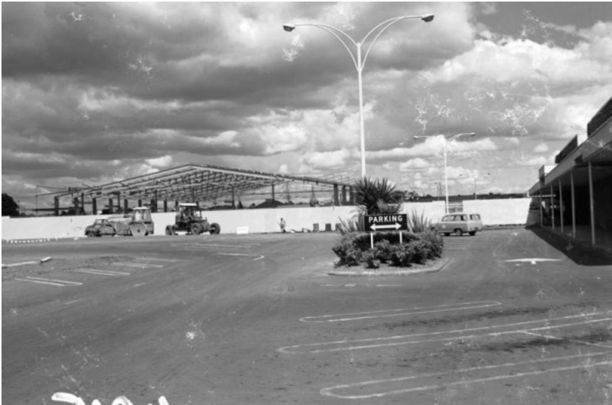
Additions to LynnMall. From Great North Road view across shopping centre parking area showing roofing framework of new structure. In front of the barricade are several of the contractor's items of heavy machinery including a grader and roller. November 1969. Image: J. T. Diamond Collection JTD-11A-04015
