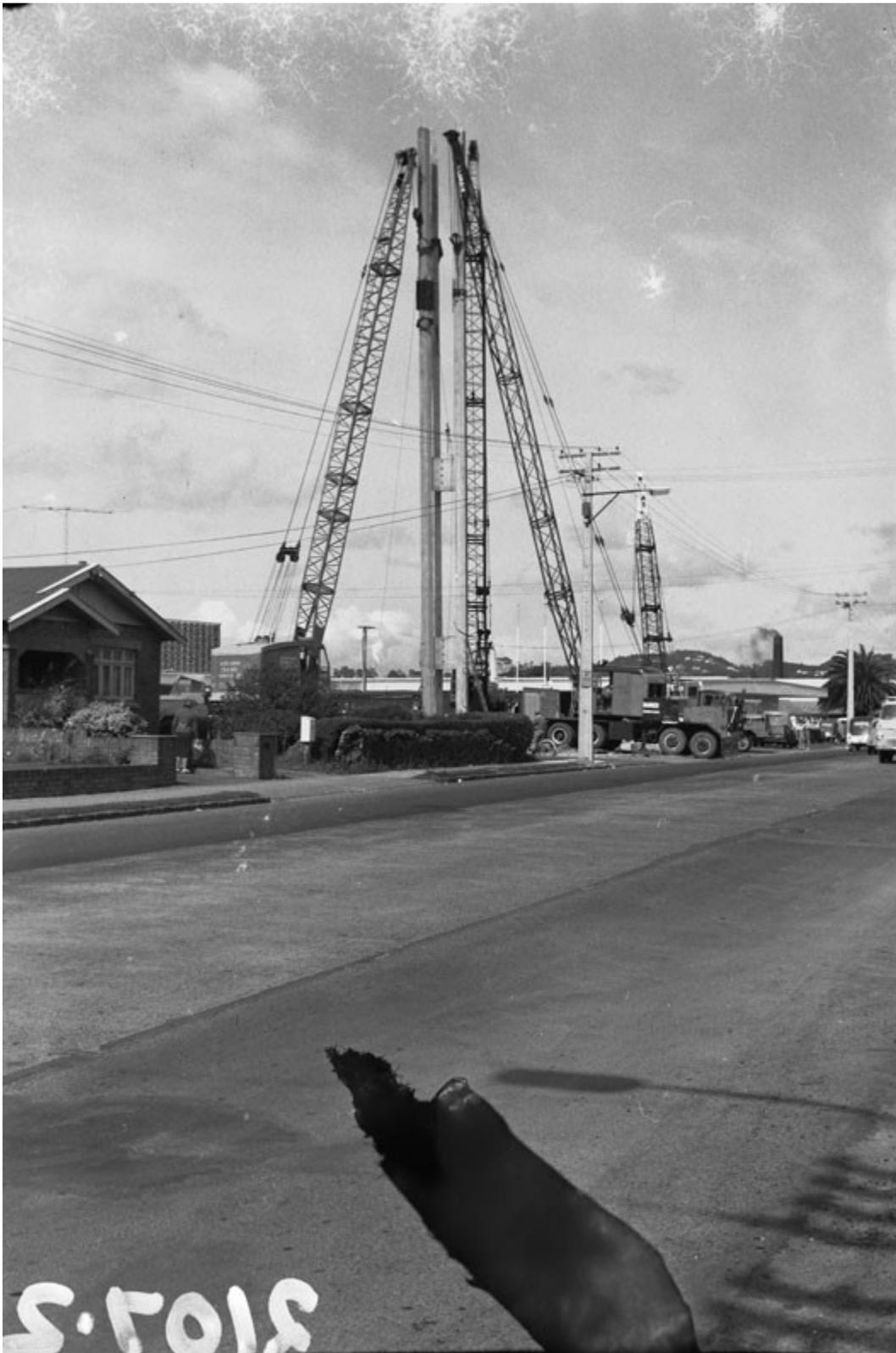
*LynnMall tower construction. View north along Great North Road showing cranes erecting a pole tower on the road frontage corner of LynnMall's car park. November 1963. Image: J. T. Diamond Collection JTD-11A-02107-2*
