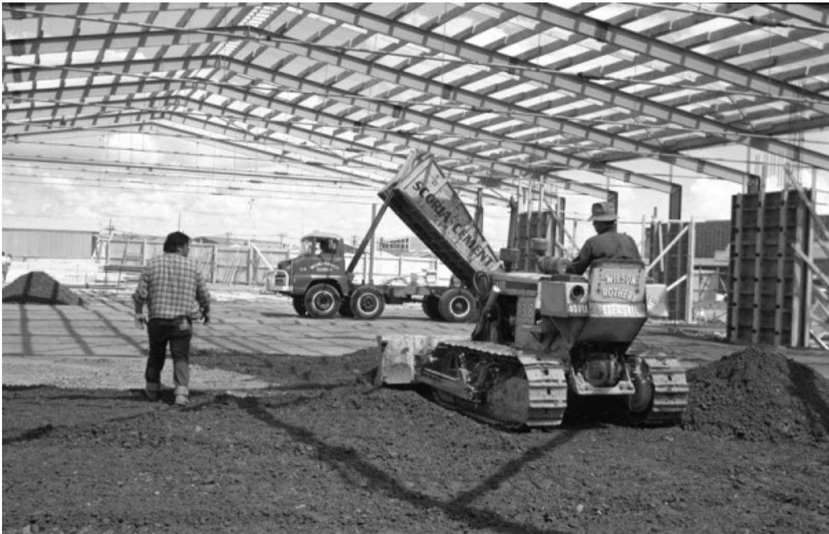
Additions to LynnMall, work in progress. Contractors at work concreting inside the new building for New Lynn's shopping mall, showing two workers, one of whom is operating a bulldozer levelling out base course beneath the girder framework of the roof with a tip truck in the background. The contractors are Wilson Rothery Ltd. of Ellerslie. November 1969. Image: J. T. Diamond Collection JTD-11A-04016-1
